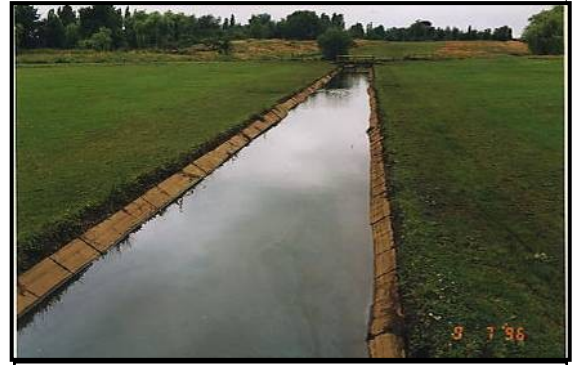
Fig 1 - The concrete lined channel of the 1970s
