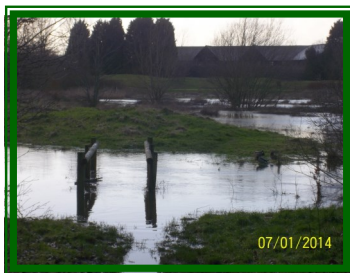
Wooden Bridge at Southwood
